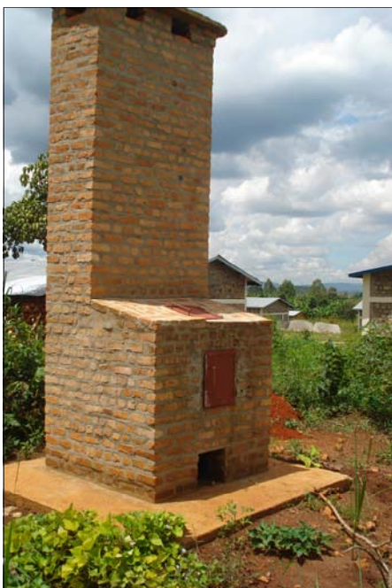
An incinerator at Nyamugari health post
